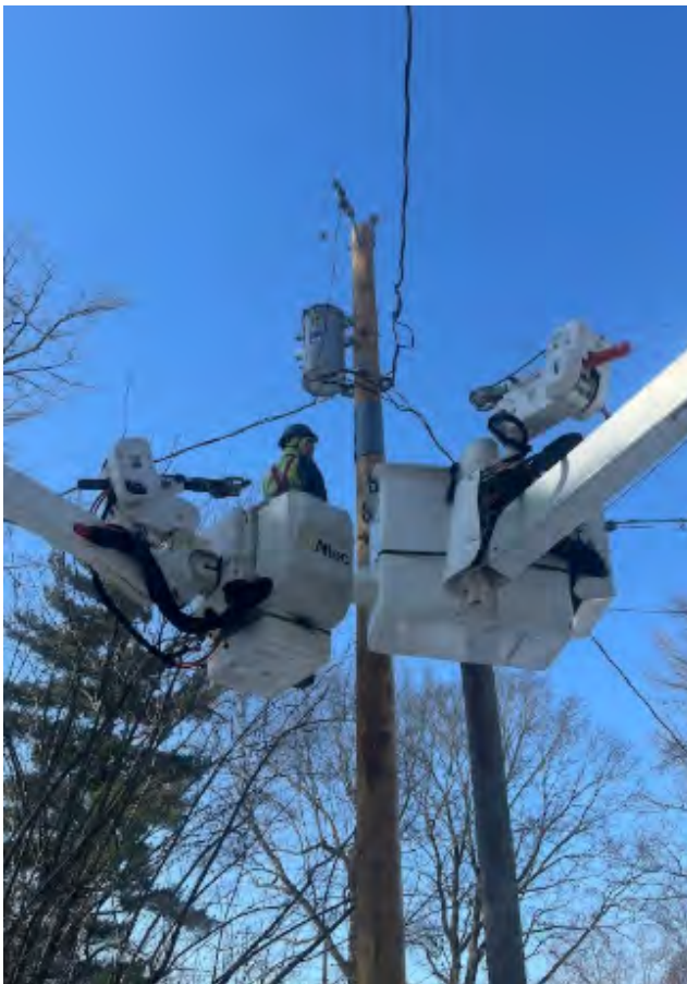
Recent Electric pole work around the village.
